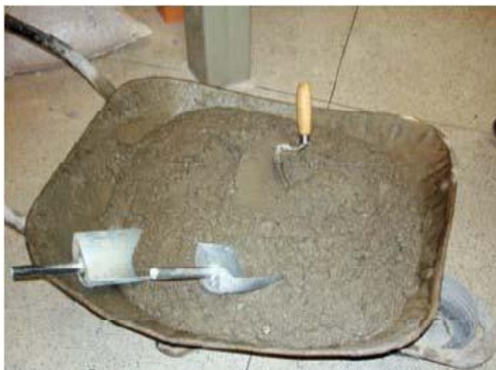
Figura 6.2 - concreto dosado (SALLES NETO, 2009)
